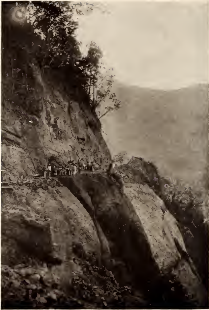
WORKING ON THE BENGUET ROAD.
